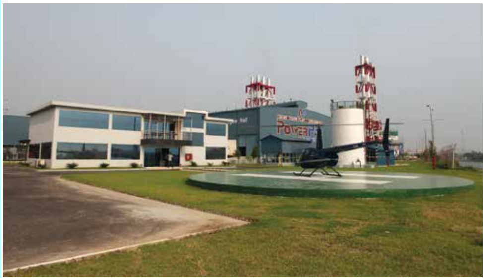
Ground View of 100 MW HFO Fired Power Plant at Keraniganj
